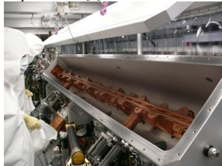
Figure 3: ReA RFQ during the final installation
